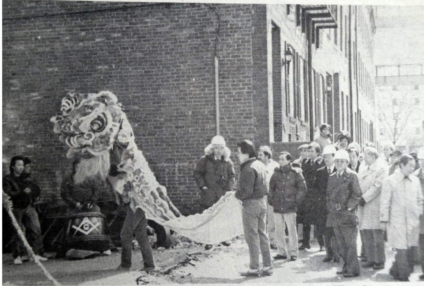
to break ground at the old Quincy School [Photo by Doris Sue Wong]
